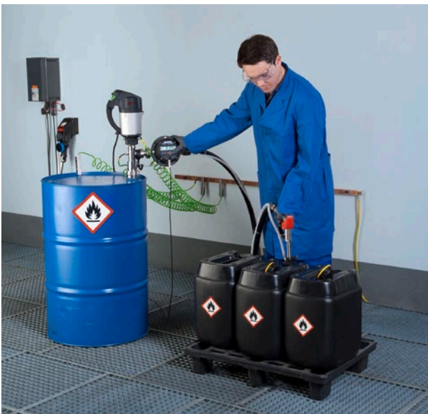
Semi-automatic canister filling in explosion zone 1.
